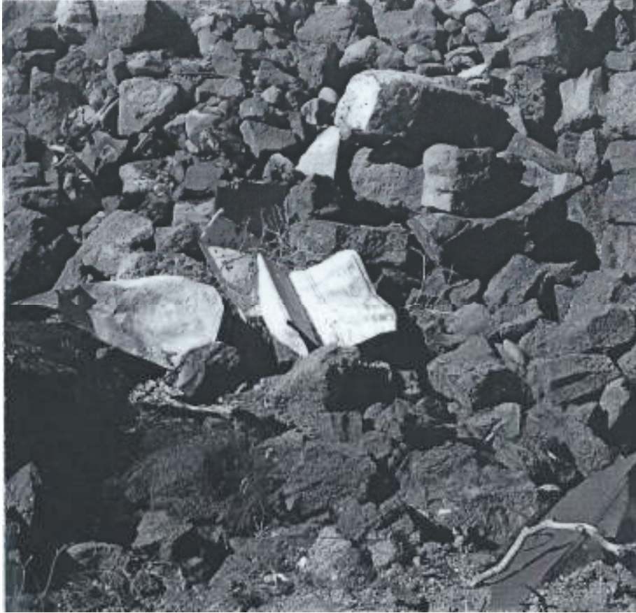
Scrap metal and cement blocks in sinkhole's rubble.
